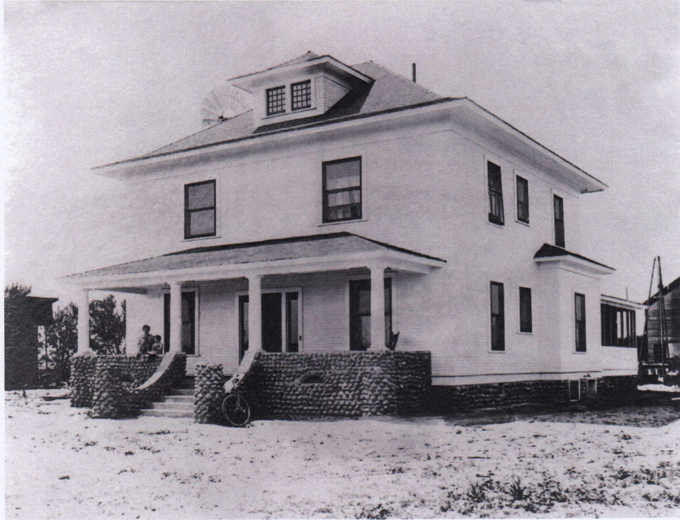
Second, and last, T. L. Reed home, built on the Home Ranch in 1908.
