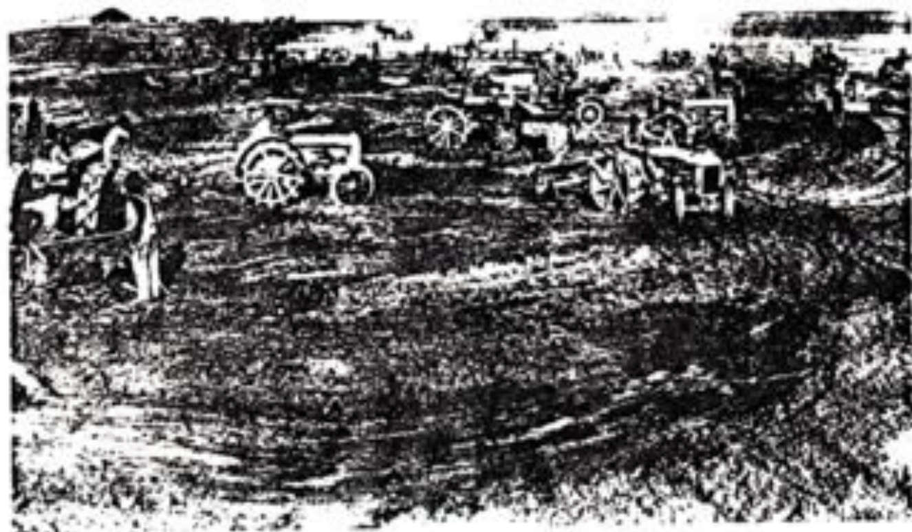
Fordson tractors till and level hogwallow.
